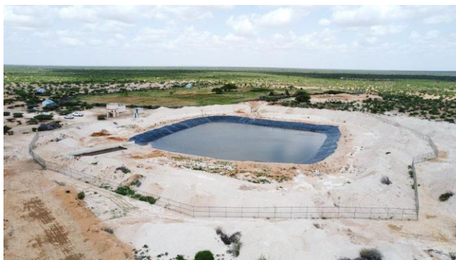
Figure 1. A haffir dam constructed by the Barwaaqo Project in Barwaaqo village (formerly Kalluun-Dacar), located 20 km outside Dhusamareeb, Galmudug. Photo/Barwaaqo Project
